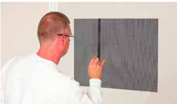
Cut down the centre of the overlap, through both layers of material taking care not to scratch the glass.
