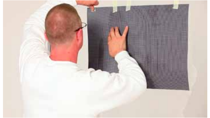
Position the second panel to overlap, align the design and fix in place.
