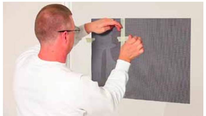
Position the second panel, aligning horizontal markers, and fix in place.
